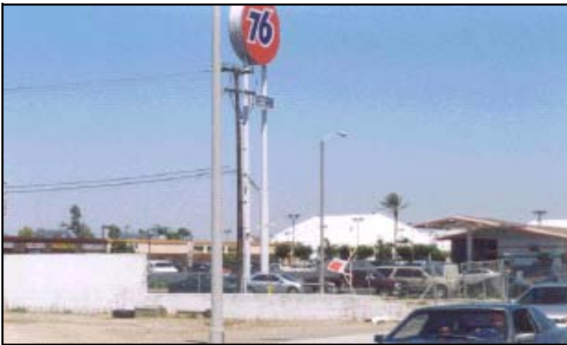
Casino under construction in 2000; bingo, barely visible, is in the strip mall to the left.
